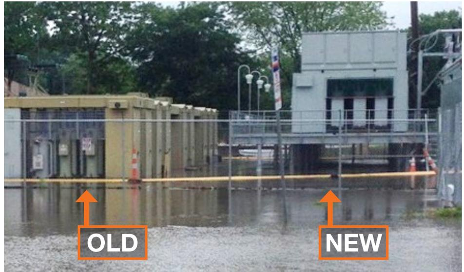
More than 4,600 PSE&G customers in Ewing and Trenton did not lose power in May 2018 thanks to Energy Strong. The program built a new, elevated station (on right) that did not flood while the lower old station (on left) flooded after storms. Now, because of work completed under the Energy Strong Program, 490,000 of PSE&G's 2 million New Jersey customers who lost power during Sandy aren't expected to lose power again due to flooding.
